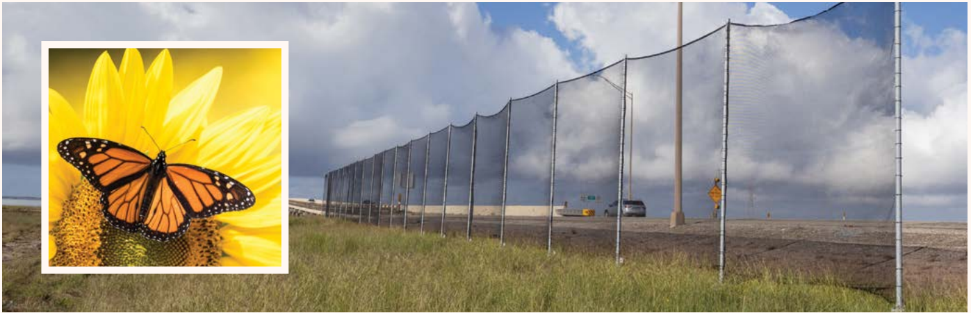
Monarch flight diverters are being tested in hopes the netting will force the butterflies to fly above the road and avoid traffic. Photo provided by Texas A&M
